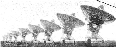
$$V(u, v) \propto \langle b_1^*(t) b_2^*(t) \rangle = F \left[ \frac{T_B(\xi, \eta) - T_{ph}}{\sqrt{1 - \xi^2 - \eta^2}} |F(\xi, \eta)|^2 \right]$$
