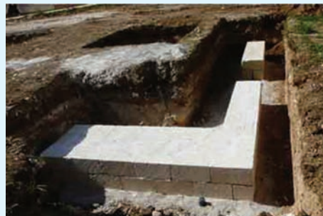
foundation walls in “Leccese” stone
