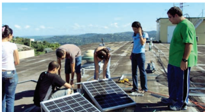
Figure 3. Students installing solar panels for operation of the OTG radar.
