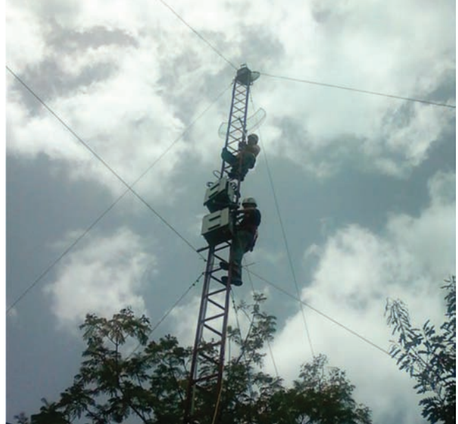
Figure 7. Students during installation of the OTG at Cornelia Hill.
